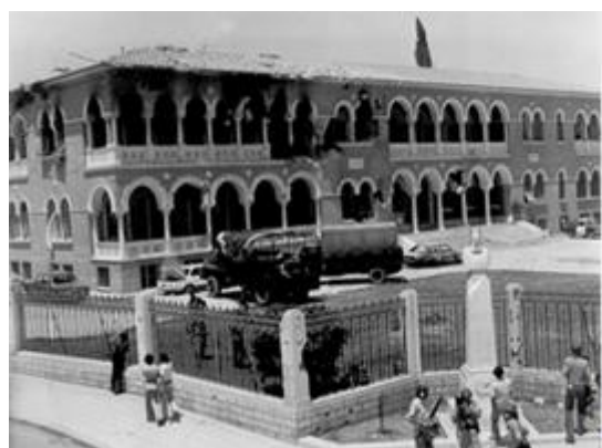
President Makarios' residence, the Archbishopric, was heavily damaged during the coup.
